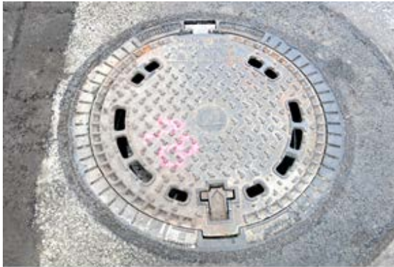
D 400 Abdeckung, Infratop (Norguss)
